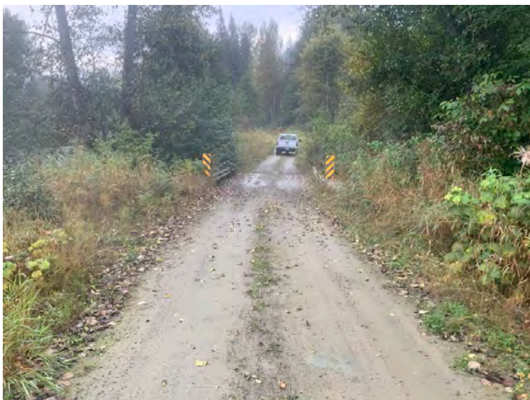
Approach from Left Bank when facing downstream
