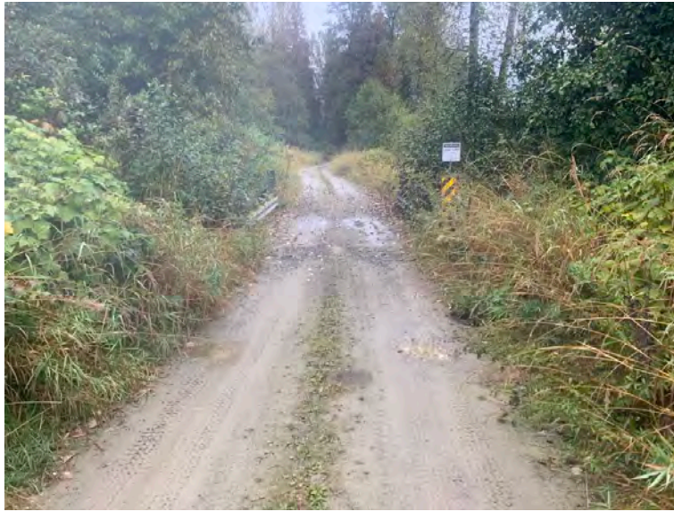
Right Bank Abutment when facing downstream
