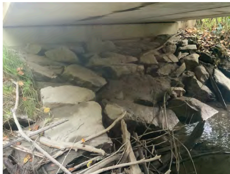
Left Bank Abutment when facing downstream
