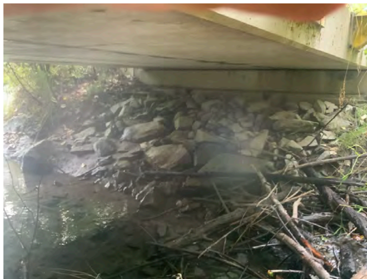
Right Bank Abutment when facing downstream
